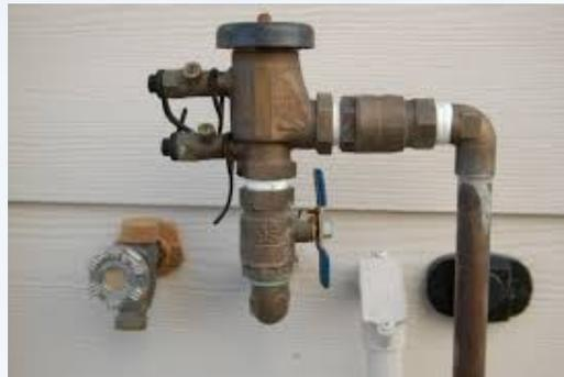
*Typical installation of a Pressure Vacuum Breaker (PVB) on a residential lawn irrigation.*
